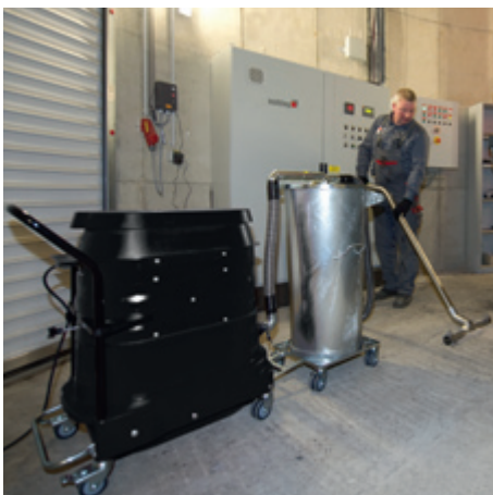
R01 A020 with pre-separator in cogeneration plant
